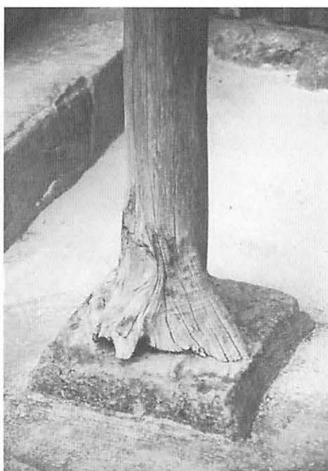
図6.5 伊是名島銘苅殿内 雨端柱
